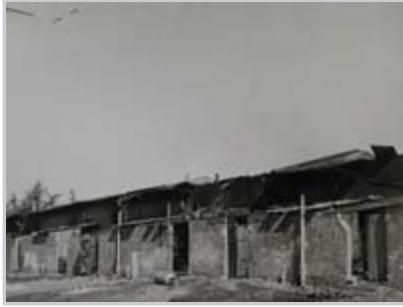
Hostel, severely damaged, Meadowlands.
