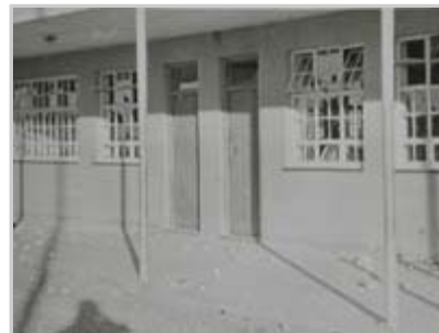
Classroom doors and windows, Mafeking school.
